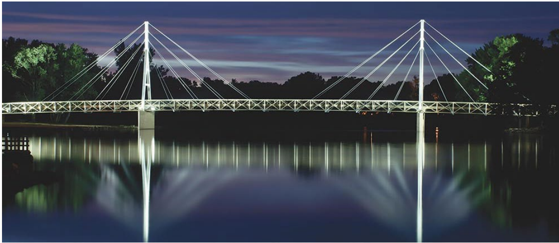
Figure 11. Example of a cable-stayed bridge
